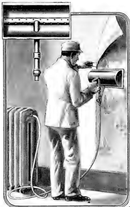
A nearby radiator supplies the steam through a hose to the apparatus in use
